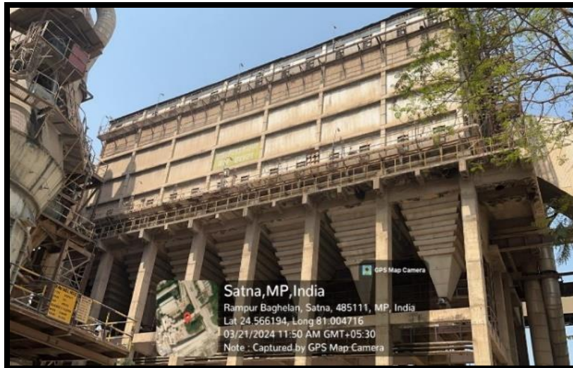
Electrostatic precipitator
